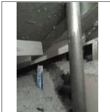
Insulation measure over 13"
