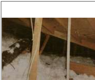
Showing insulation and attic roof structure
