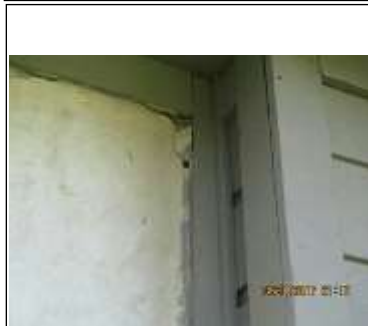
Small hairline crack repair under window in dining room
