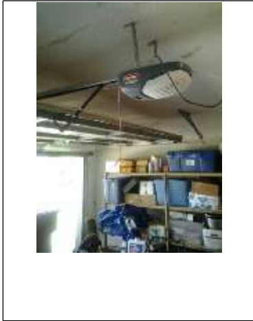
Manuel lock operational. Should be bolted to prevent lock from being used
