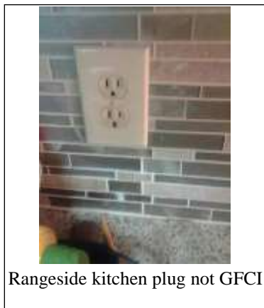
Range side plug2 not GFCI
