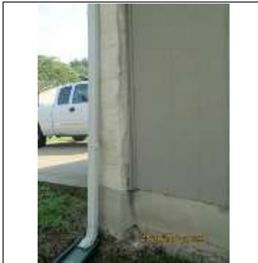
Damaged downspouts
