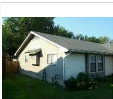
Larger view of roof
